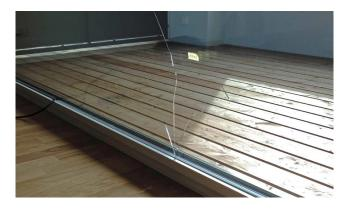
In sliding door systems with heat and sun protection glass, direct sunlight can cause heat build-up between the panes when they are slotted one behind the other when open, which can also cause thermal shock. The same problem often arises with infrared-reflecting blinds or curtains with insufficient air circulation.
