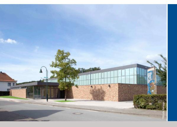
of synthetic hollow fibres lies between fibre glass mats, which transmits the incident light and diffuses it evenly. The capillary slabs minimise the solar gain and prevents convection in the glass. Besides reducing the cooling loads in the building, the Ug-value of the façade is improved significantly, which saves precious energy. The good colour reproduction of the insulating glazing can also be discerned
